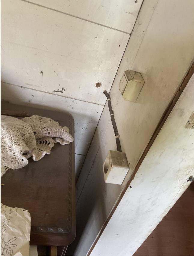
A photograph showing a close-up of electrical wiring on a wall. The wall is made of light-colored panels, some of which appear to be non-fireproof. Two electrical boxes are visible, one above the other, connected by a dark cable. The wiring is not properly secured or protected, and there is a visible gap or break in the grounding continuity. A brown leather chair with a white lace cloth draped over it is partially visible in the foreground on the left. |
